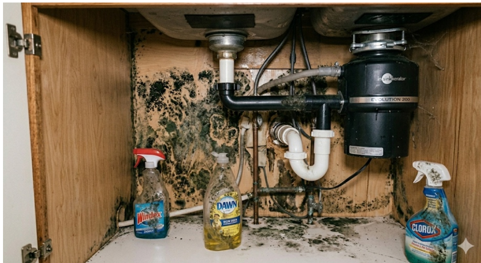
Mold colonisation can begin within 24–72 hours of a moisture event on any organic surface.
